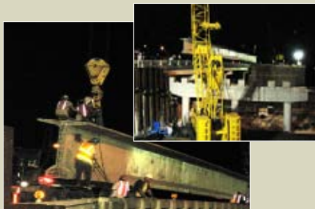
Beam setting at Commercial Blvd
