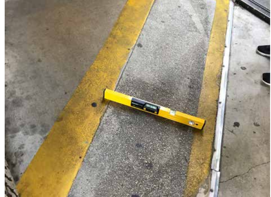
Figure 5.1: ADA assessment team using smart-level to measure ramp slope.
