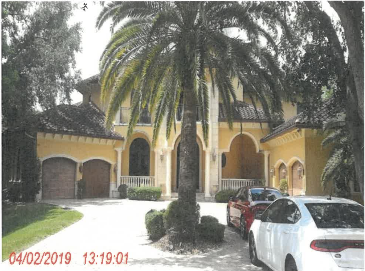
Figure B-2 – On-site conditions
