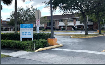
Image: Study Area Office Bldg. (4100 NW 3rd Ct)
